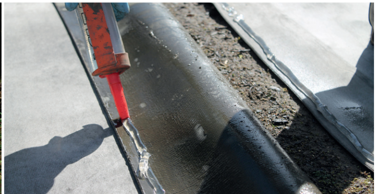
Double cordon de mastic
