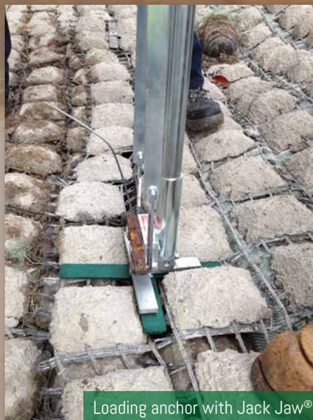
Gas powered driver installation.
