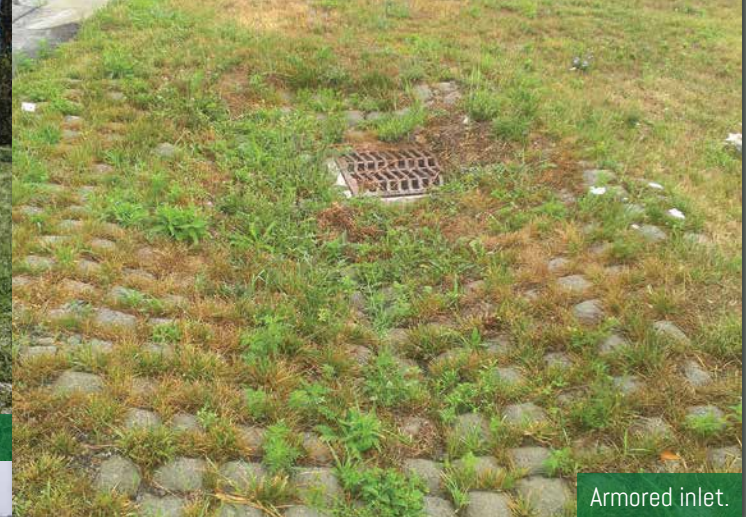
Outlet armored with Flexamat®, 3 years after installation.
